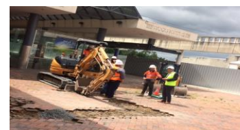
Next phase of demolition has commenced
